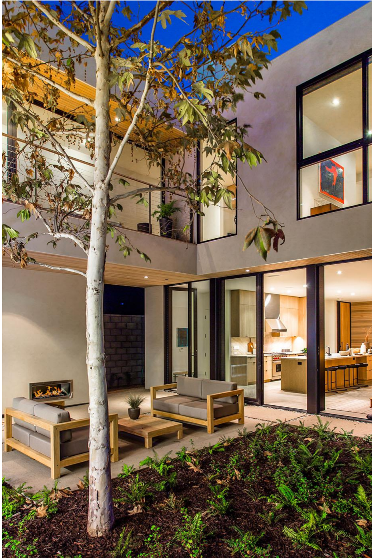
Award-winning architects Marmol Radziner's newest collaboration with Halton Pardee is this $4.775 million listing at 613 Santa Clara in Venice.
